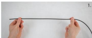
1. Measure the desired cable length and add approx. 6 cm / 2 1/2" that will go inside of the connectors on either side.
