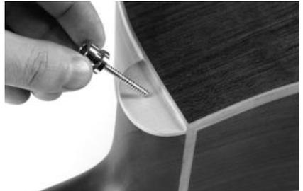
Install the strap lock only at the neck point, which is strong enough to hold the screw. Drill a hole with a 2mm wood drill first.
